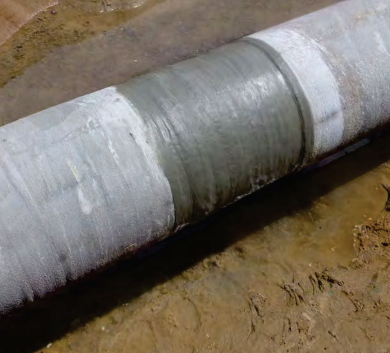
Welded Joint 20 in (500 mm)
