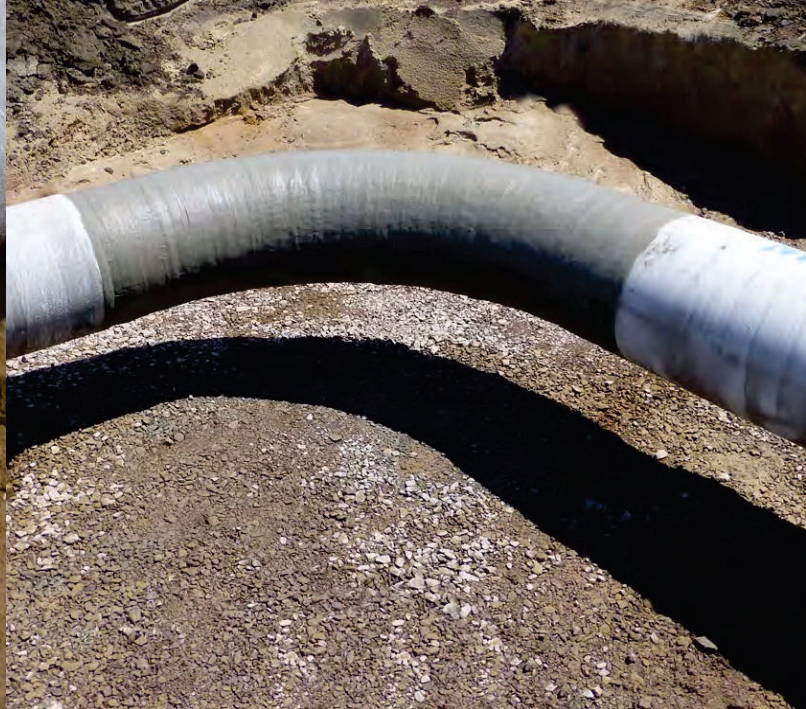
Pipe Elbow 20 in (500 mm) D5 90°
