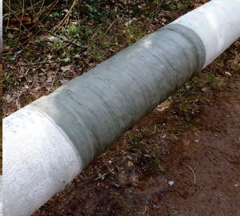
Welded Joint 6 in (150 mm)
